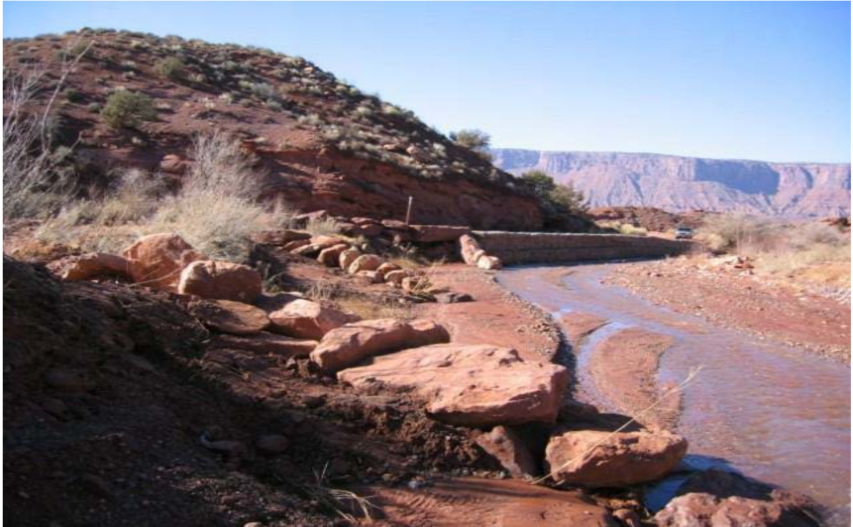
Figure 16 – Large rock barbs in foreground, gabion baskets in background
