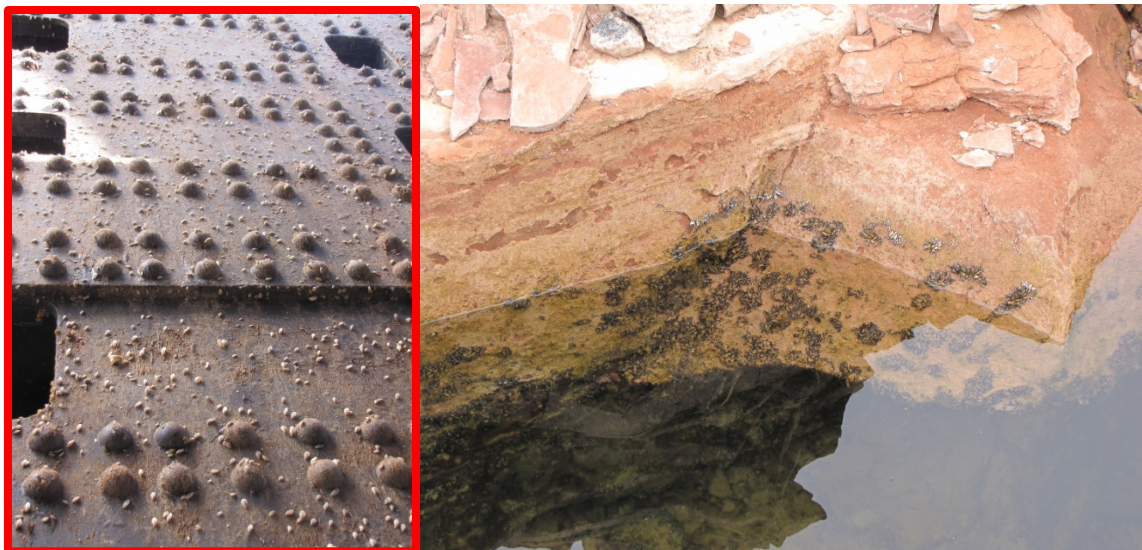
Figure 36- Wheel gate from Glen Canyon Dam and rock wall with mussels.
